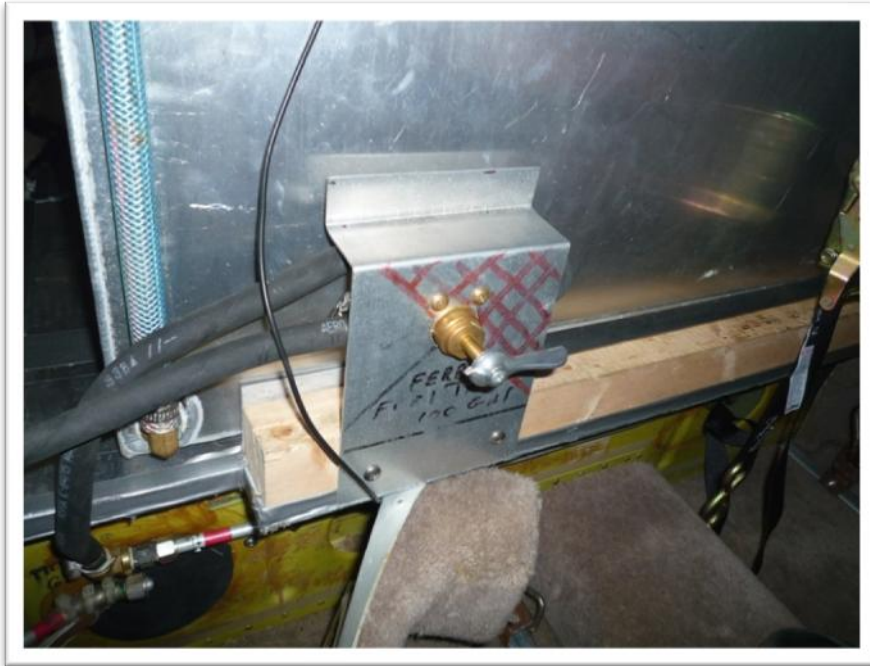
Fig. 11 The lever auxiliary fuel cock in the position when the right wing tank was connected only with the auxiliary tank
